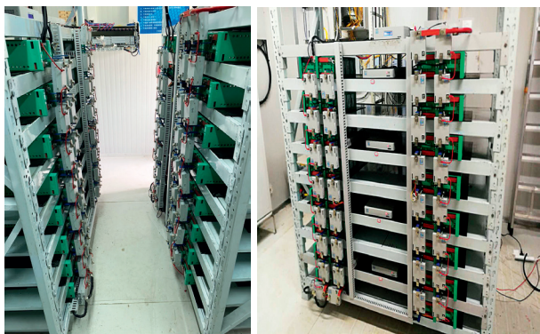
图6 通信基站数字无损梯次利用储能系统应用部署 Fig 6 Deployment of DES in communications base station
