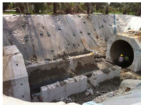
Fig5 Pipe Cutting and Connection Renovation
